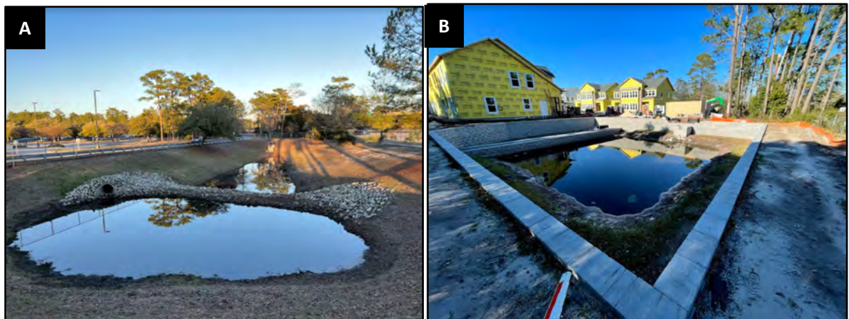
Figure 1. Design Fundamental: Inlet structure angled away from forebay berm, and well armored berms. A. Flared end section with energy dissipators to reduce scour. Forebay with protected internal flow path – berm side slope – armor. B. Well armored forebay with concrete walls protecting the internal flow path.
